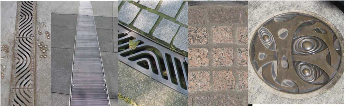
Expressive drain covers are elements that give interest to the ground plane.
