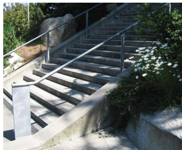
Handrail leading down Fisher steps is simple and modern.
